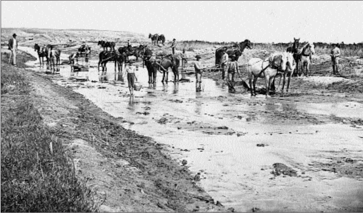
Construction of the mammoth Eureka irrigation canal in Ford County (left).
