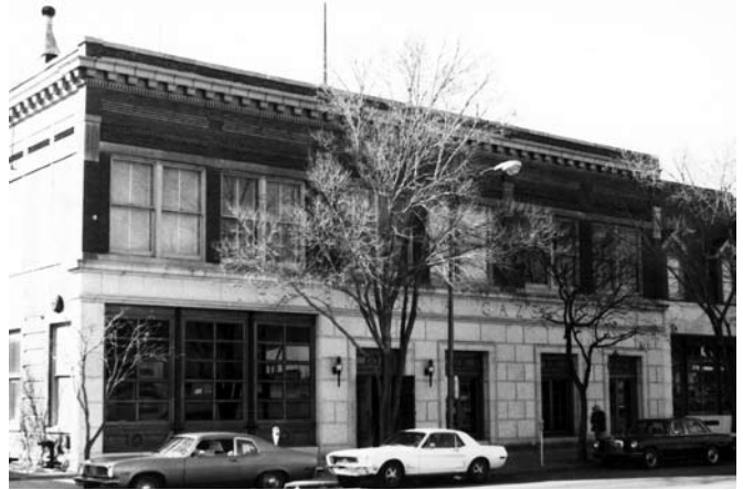
In 1895 William Allen White bought the Gazette with borrowed money. By 1900 the paper was well established enough that White was able to build the two-story structure that still houses the paper today at 517 Merchant Street in Emporia. Pictured here are the paper's offices after their 1967 renovation by W. L. and Kathrine White, with what is likely Call's white Ford Mustang parked out front.
