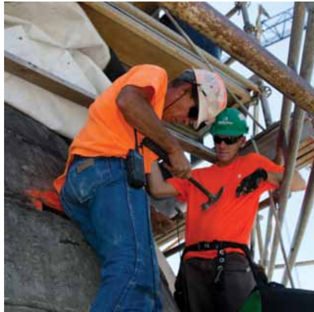
Workers install new copper on the Capitol dome as part of the multiyear restoration.
